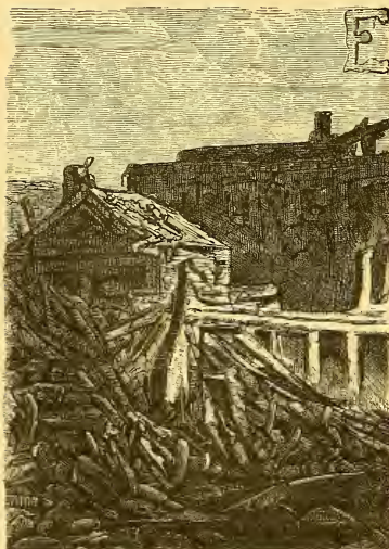
AFTER THE EARTHQUAKE.
